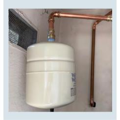
Determine pipe insulation needs between the tank and building envelope.
