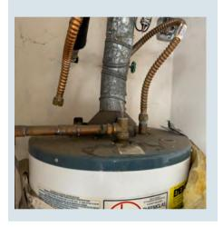
Drain the tank, using a transfer pump if needed.
