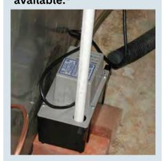
Install a T-fitting on the condensate outlet, or a T with a removable cap to allow for cleaning.
