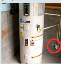
Ensure the condensate drain's diameter matches manufacturer specs with at least 1/8" per foot slope.
